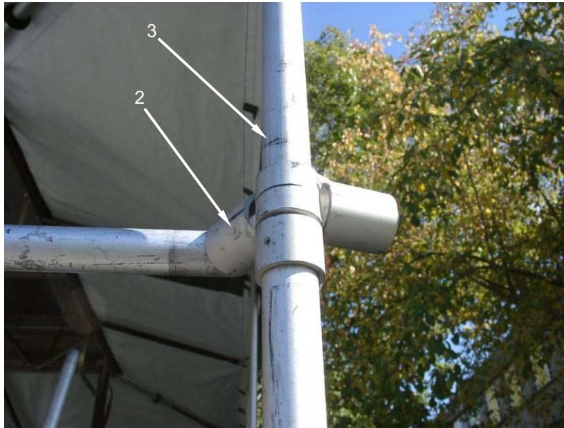
Locate and install screen assemblies (1) by matching the letters at the top corners of the screens (1) to the letters on the roof canopy flap (2). Hook and pile fastener (3) is used throughout the fabric installation to reduce setup time. Stretch fabric sections together in correct position to each other. Press hook and pile fasteners (3) together firmly to secure.
