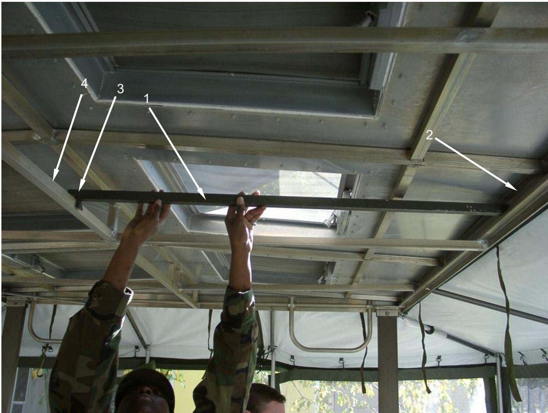
Hang the exhaust fan assembly (1) on the prop rod (2) by engaging the hook-shaped bracket (3) over the prop rod (2).
