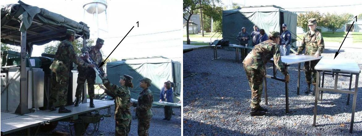
Loosen cabinet and dispenser straps (1). Remove strap assemblies and set aside.
