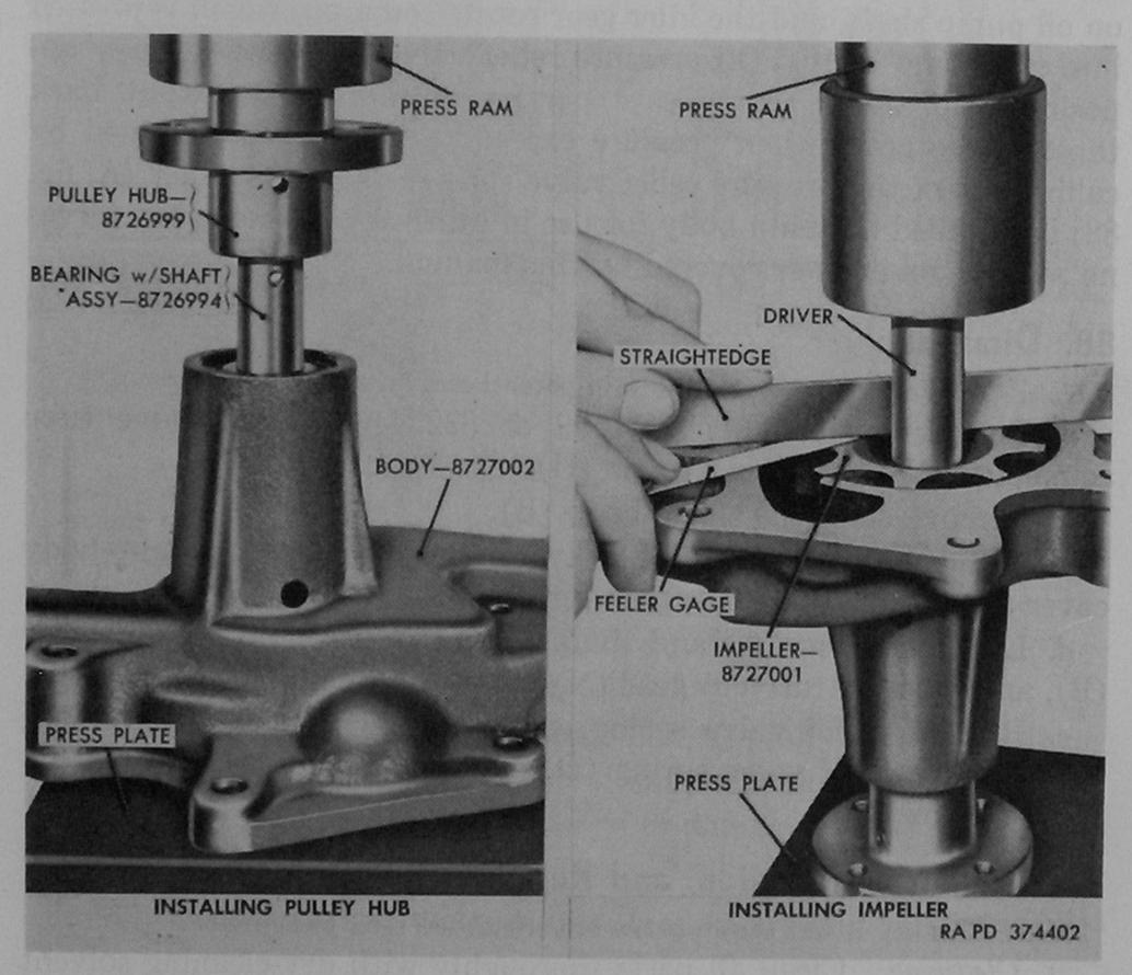
Figure 87. Installing water pump pulley and impeller-engine assembly 8726920.
