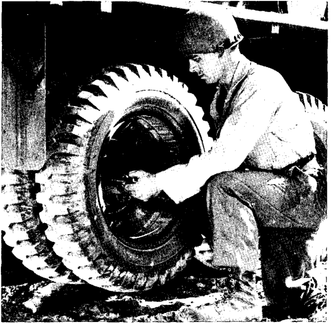
Figure 58. Substitute for a jack to remove outside dual wheel.
