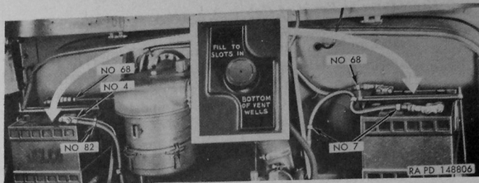
Figure 44. Battery cables installed.
