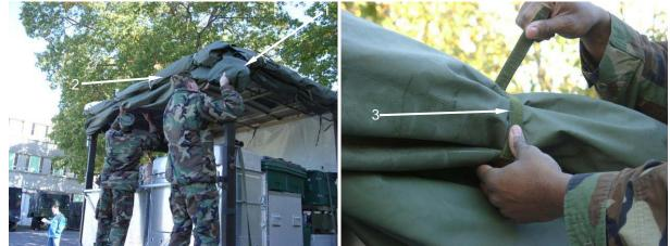
Retrieve the roof jacks (1) from their storage location and set the pawl (2) to the latching position.
