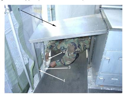
Remove fabric holdout struts (if used), and set aside.
