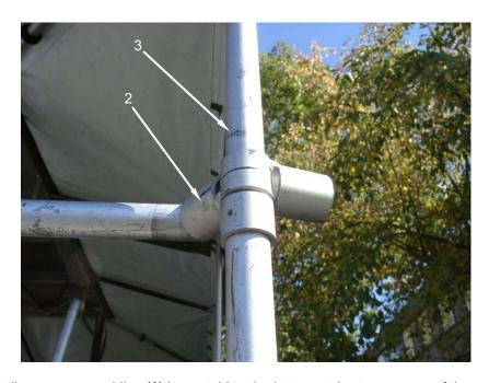
Locate and install screen assemblies (1) by matching the letters at the top corners of the screens (1) to the letters on the roof canopy flap (2). Hook and pile fastener (3) is used throughout the fabric installation to reduce setup time. Stretch fabric sections together in correct position to each other. Press hook and pile fasteners (3) together firmly to secure.
