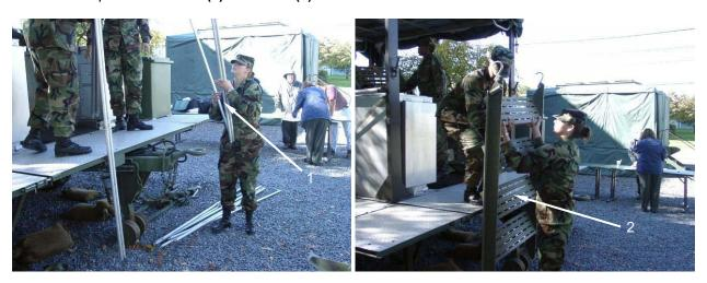
Install three ladders (1) and handrails (2) onto ramps at entry and exit. Engage the hooks (3) at the end of the ladder (1) into the holes (4) on the ramps (5). There are nine possible locations for the ladders (1). Install two handrails (2) on each ladder by engaging the ends of the handrails into the receptacles (6) in the ladder (1).
