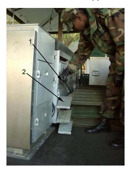
Remove roof canopy supports (1) and stow along the floor on the left and right side of the ladders (2).
